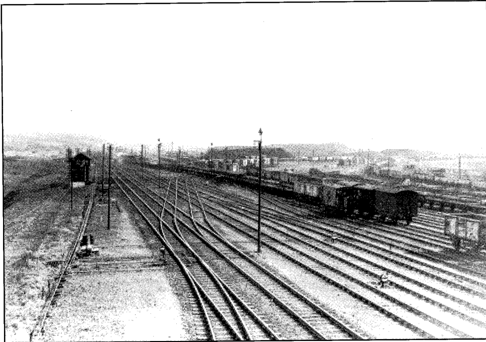
Frodingham Trent Sidings looking towards North Lines Junction c. 1960. John Oxley.
